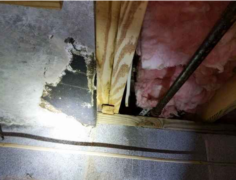
4 - below the chimney
