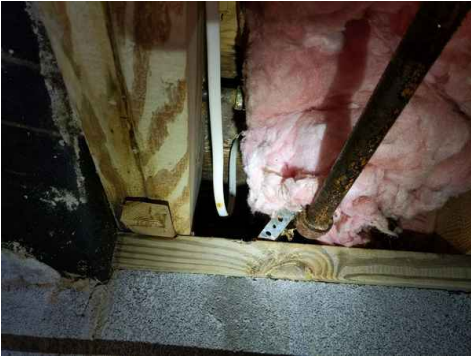
4 - below the chimney
